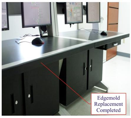
After removing existing Edgemold use care when scraping off old epoxy to avoid damage to paint; "touch up" paint is available in parts list on next page
